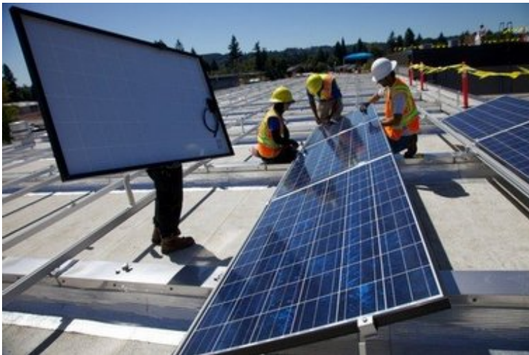
Installing panels on Gladstone High School in Gladstone, Oregon.
