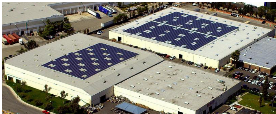
A 743 kilo-watt Solar System in City of Industry. Using only a portion of the available roof, this system brought the owner's electricity bill to zero.
