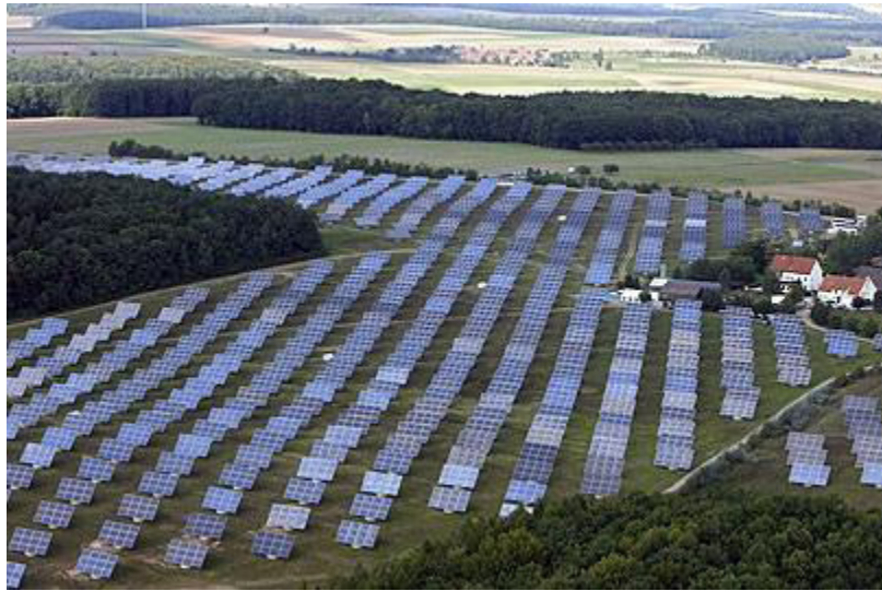
A solar farm in Perth, Ontario
