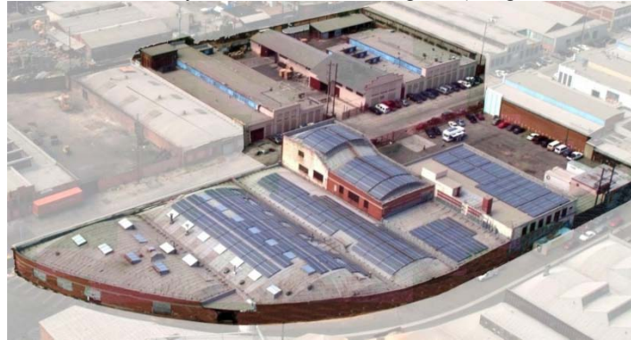
Figure 6: A 225 Kilowatt System in South Los Angeles (Image source: Kahn Solar)
